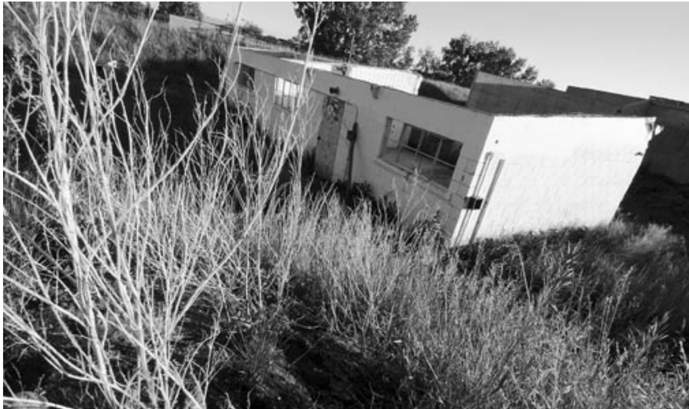
Derelict building at Griesbach Barracks, in north Edmonton.
